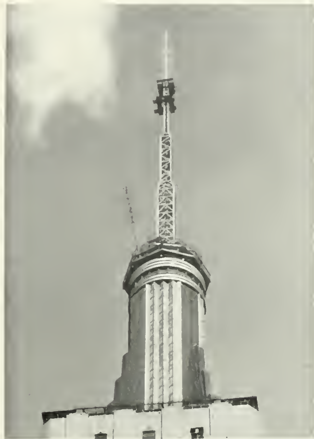
Station WNBT recently began regular transmissions from the new 215-foot television mast atop the Empire State Building.
